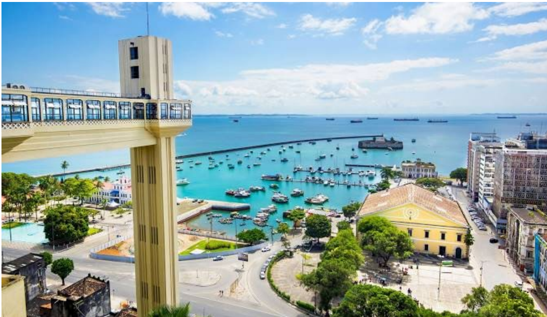
Lacerda Elevator connecting the lower and upper city neighborhoods
